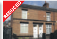
Windleshaw Road, Dentons Green
